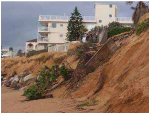
Coastal erosion at Collaroy/Narrabeen beach
